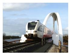
Fig 8 -- The completed Bert Swart Bridge across the Van Starkenborgh Canal in Zuidhorn, the Netherlands, handles two passenger trains per hour on weekdays, as well as freight traffic as needed. The 200-meter long 1,700-ton steel bridge blends architectural beauty and strength. The Xypex-coated concrete rail bed will lower mainenance costs and extend the life of the bridge.
