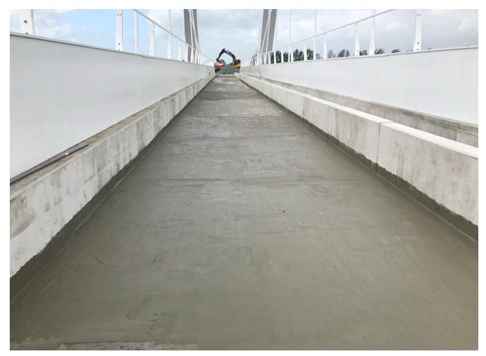
Fig 7 -- Xypex Conentrate has been applied to the concrete deck of the new Zuidhorn railway bridge, creating a integral bond and protect the concrete from moisture and harsh chemicals.
