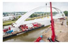
Fig 2 -- As assortment of heavy lift technology is employed by the Mammoet company in order to move one end of the 1,700-ton steel bridge across the canal and into its final position.
