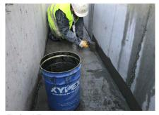
Fig 6 -- A Totech technician applies Xypex Concentrate with a stiff bristle brush along a walkway incorporated into the new Zuidhorn railway bridge.
